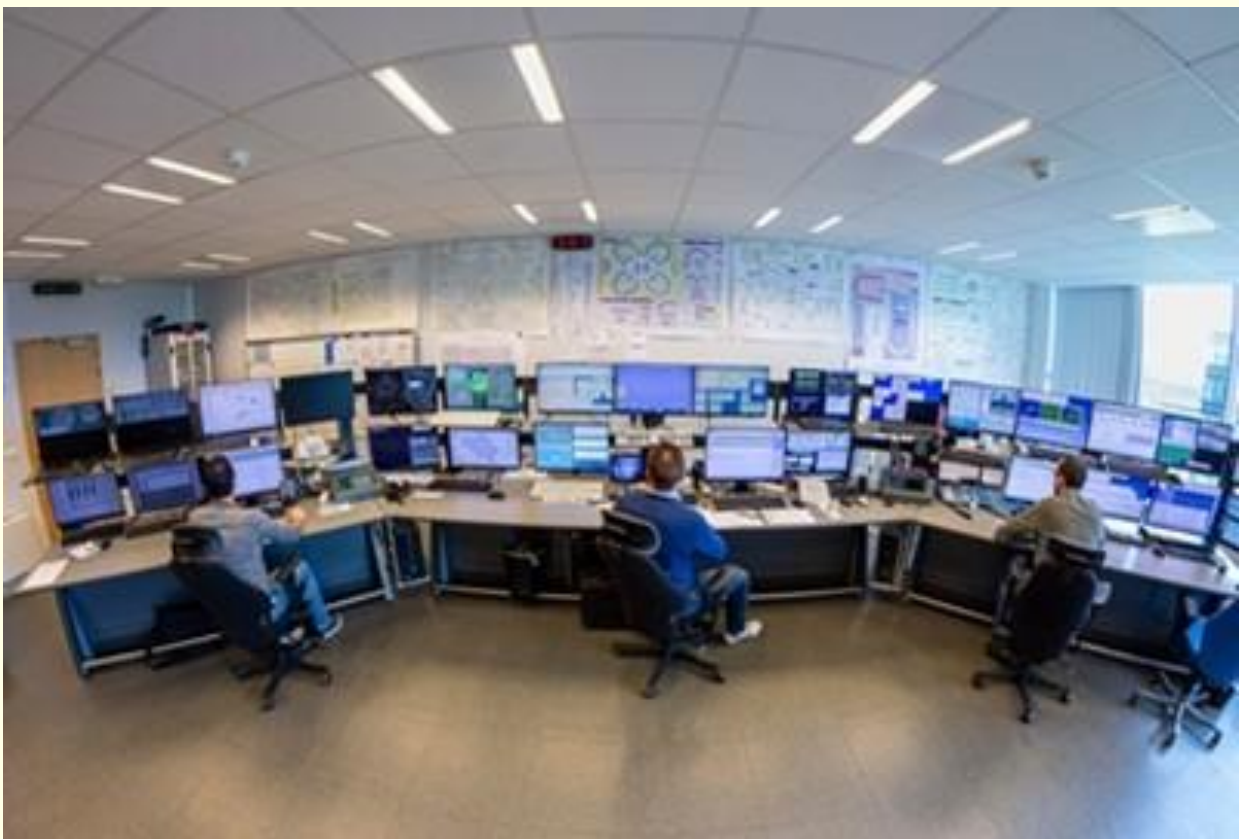
Image 11 ATSEP Working positions for Systems monitoring and Control
